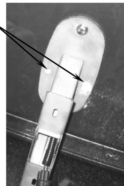
9. Remove brackets from roof and apply a generous amount of supplied silicone into and around all bracket-mounting holes.
